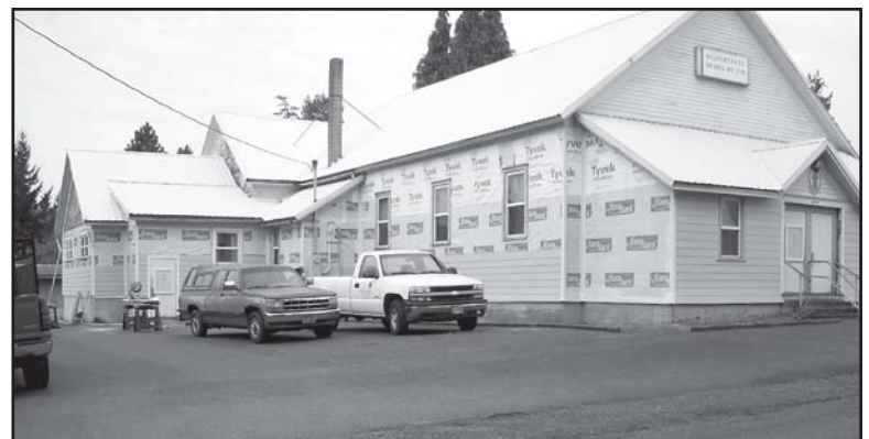
New Hardy Plank Siding being installed on Beavercreek Grange #276
