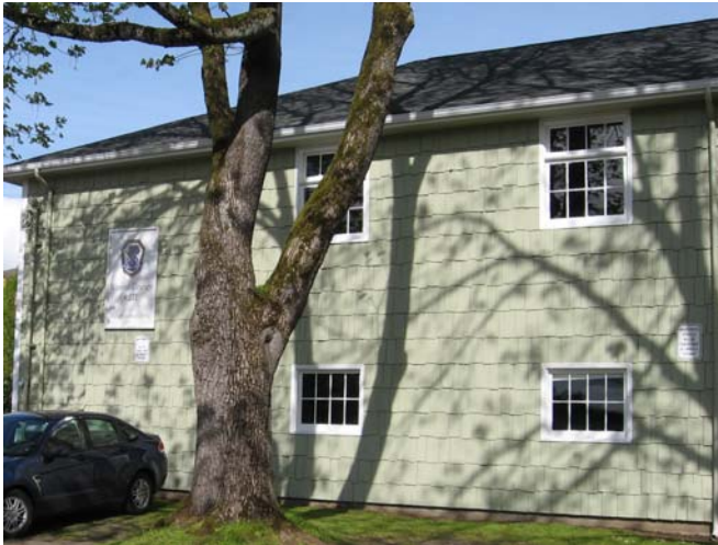
The new paint job and light green color spruced up the exterior our historic building.
